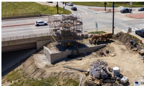
Castle Pines Parkway Gateway Monument under construction
