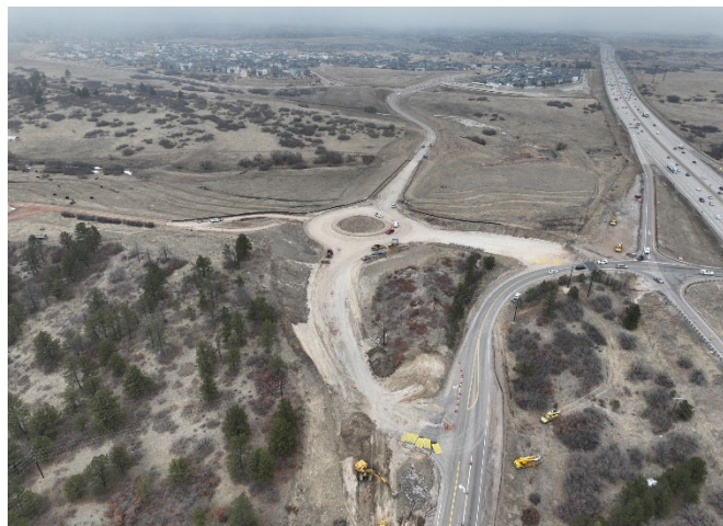
Lagae Road round-about under construction
