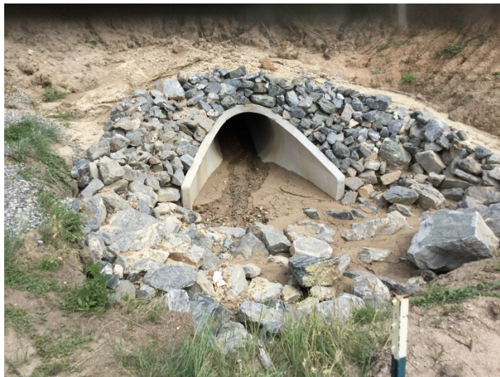
Stormwater Drainage Outfall
