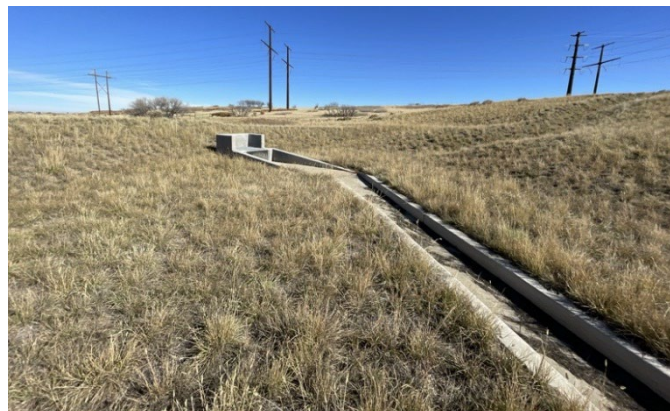
Stormwater Extended Detention Basin with Trickle Channel leading to Outlet Structure
