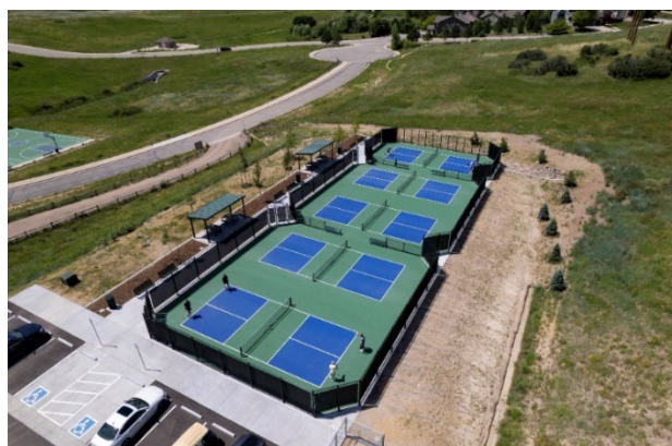
Pickle Ball Courts completed in 2023 at Coyote Ridge Park
