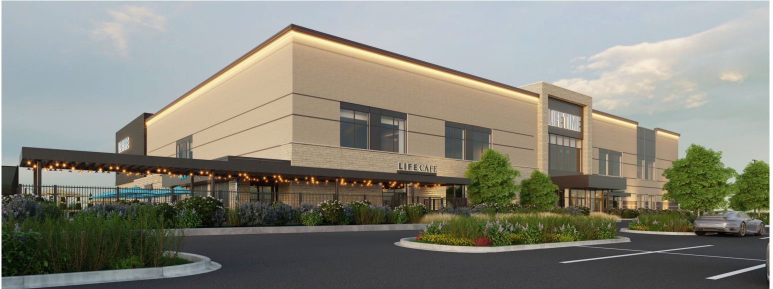
A new Life Time facility is currently under construction. The facility is currently scheduled to open in late 2026.
