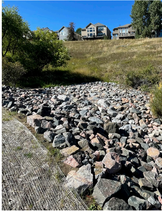
Before and after photos of stormwater drainage improvements to the Daniels Park Pond cutoff wall.
