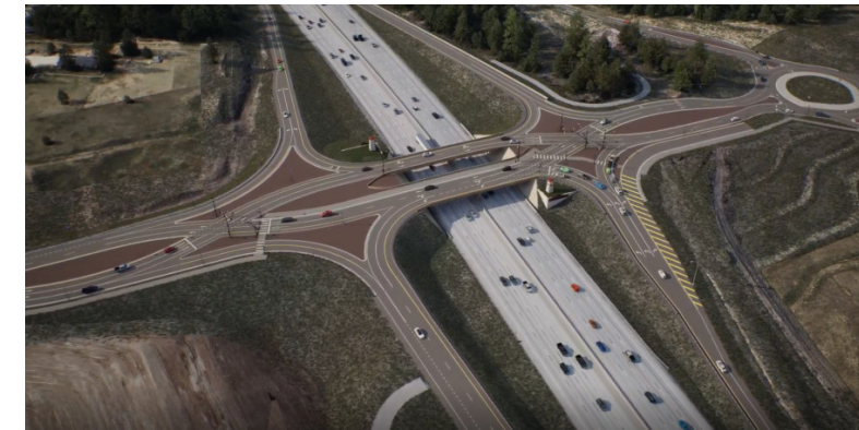
Rendering of the diverging diamond interchange that will replace the current layout of the Happy Canyon and I-25 interchange during the reconstruction project.
